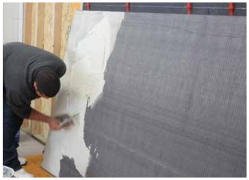
• Large porcelain panels can be installed over concrete or other suitable substrates. You must honor all expansion joints or any defects in the substrate and mitigate prior to installation.
