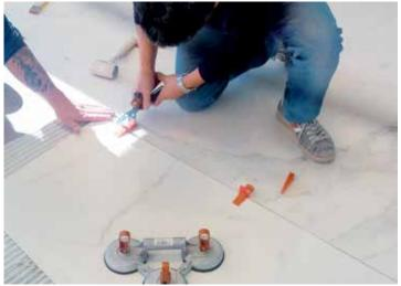
• Self-leveling systems are required to acheive desired flatness between joints. Fill any voids with the mortar for complete support.
