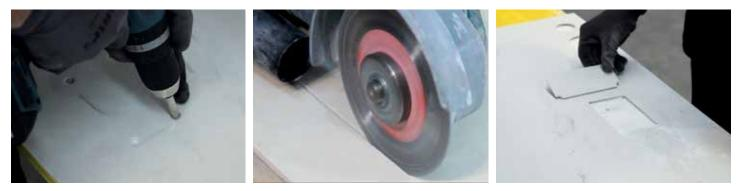
• When possible, it is best to fabricate niches and holes after the panel is already installed with thin set on wall or floor. If it is not possible to cut holes or square/rectangular cuts (fireplace, sink, etc.) before the panel is installed, create full support with plywood or MDF panel template with same shapes and cuts to attach and transport the porcelain panel. Support panels should only be detached when porcelain panels are fully bonded to the substrate.
