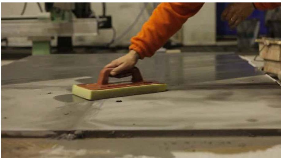
To do this correctly, you should plaster and wipe a surface of 10m<sup>2</sup> maximum at a time. When plastering rough flooring sandblasted, flamed, bush-hammered, antique use the same procedure.
