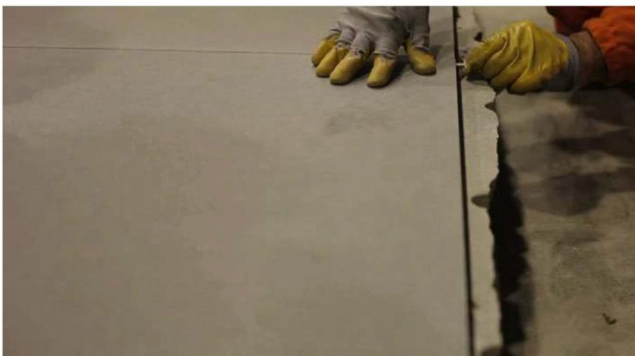
Before starting the pre-treatment, remove any traces of glue from the surface as soon as possible using a dampened sponge.
