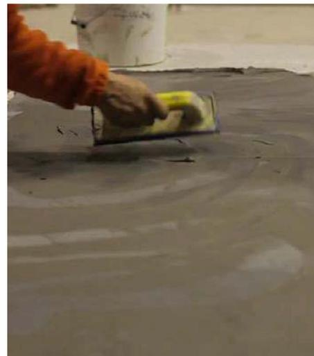
Once the product has started to dry, clean the surface with a slightly dampened rigid sponge using circular movements.
