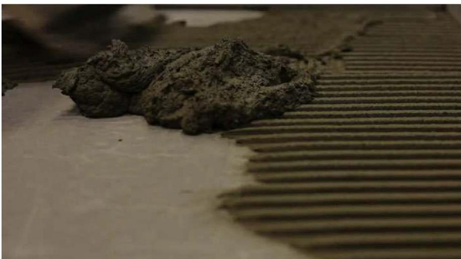
In areas larger than 40x40cm also spread adhesive on the back of the slab making sure that it is completely covered.
