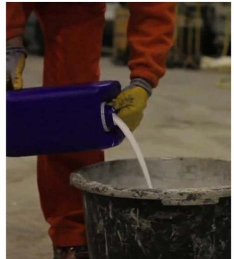
The paste will remain usable for 45 minutes at a temperature of about 23 °C, while higher temperatures will reduce this length of time.
