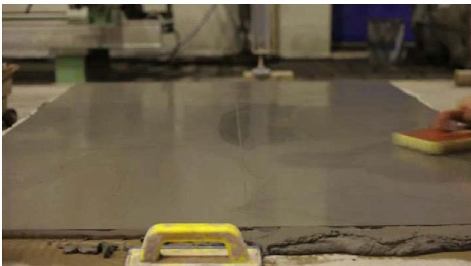
With a clean sponge, completely remove excess plaster in single, parallel movements, taking care to rinse out the sponge after each wipe.
