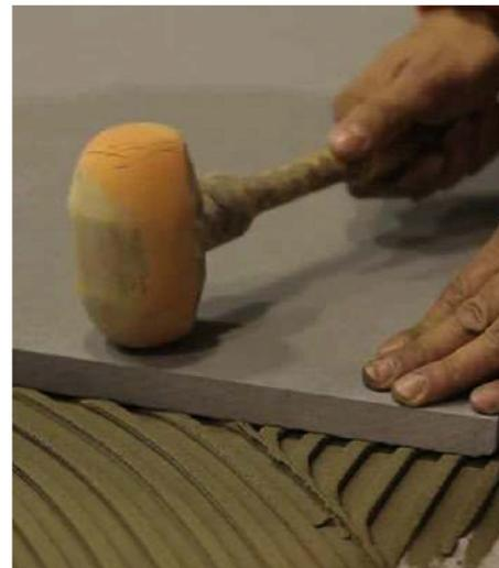
To lay the slabs correctly, use cross or T spacers. The surface can be walked on after about 4 hours, and will be fully usable after 24 hours.
